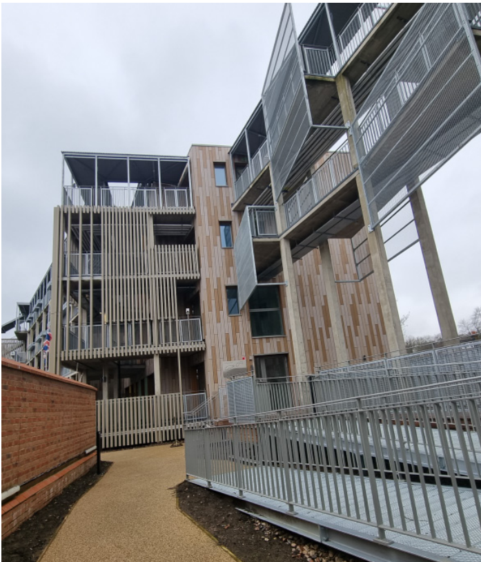
Church Grove housing project
